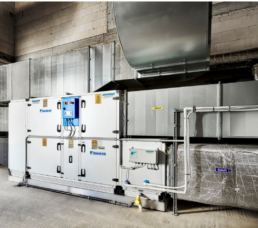
D-AHU Modular R installation
